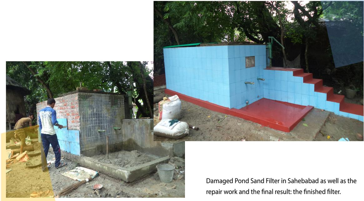
Damaged Pond Sand Filter in Sahebabad as well as the repair work and the final result: the finished filter.
